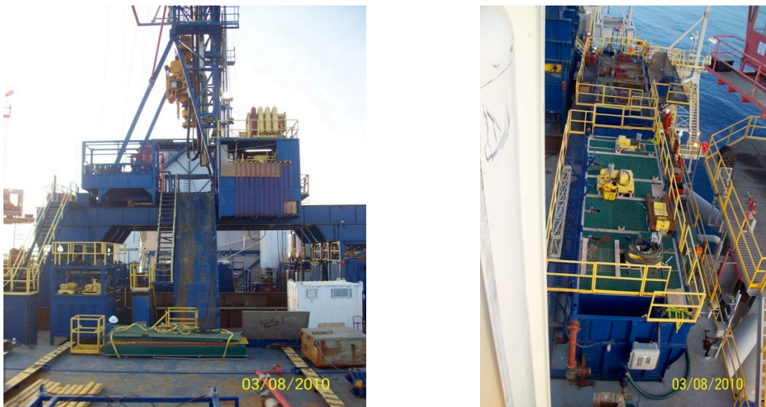
Figure 15 – Platform Workover / Drilling Rig on Mari-B Platform
